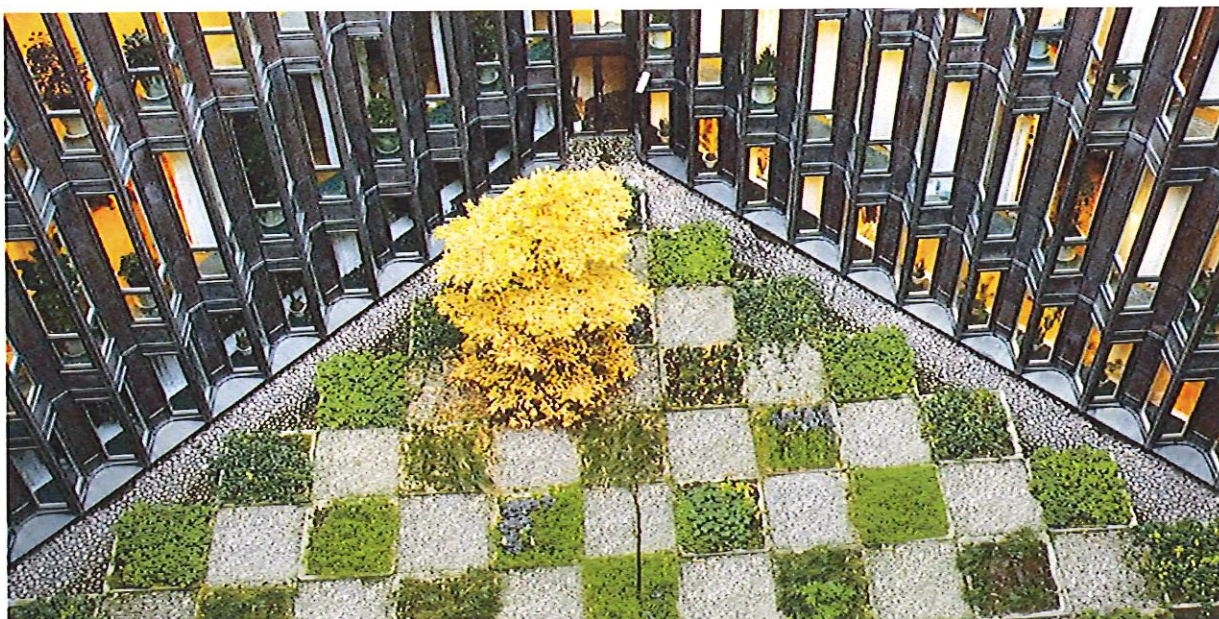
The courtyard is square in form and paved in chequerboard pattern, with alternating stone paving and plants.
